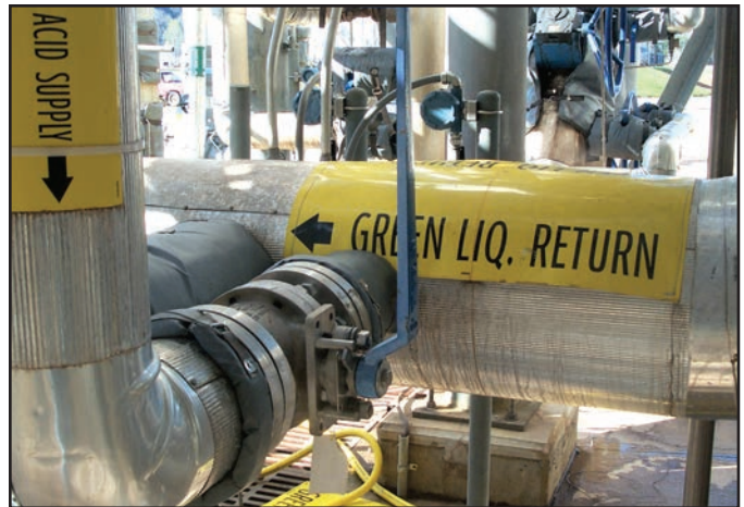
Split-body ball valve in pulp and paper.
