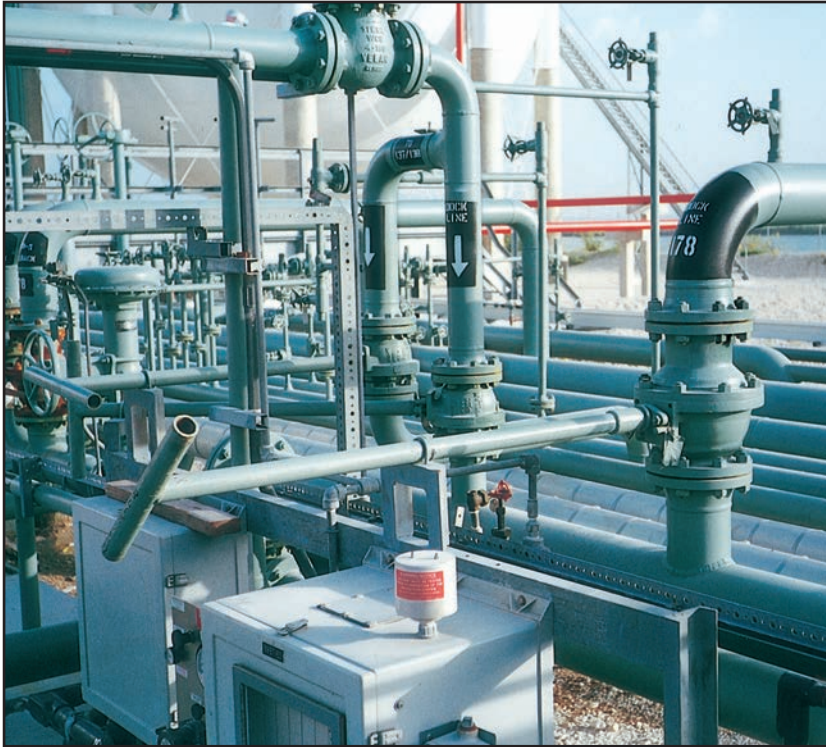
Installation of 6" SB-150 with extension handle at a Texas refinery.
