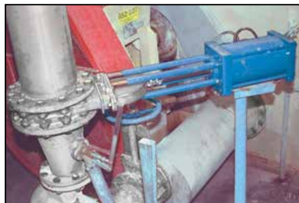
Pump discharge shutoff 5% pulp at 70 psi (4.8 bar) cycling over 75 times a day.
