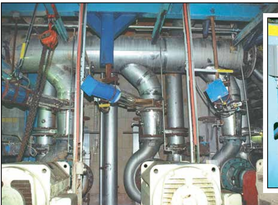
Multiple pump discharge isolation with pressure 70-90 psi (4.8-6.2 bar) white water.
