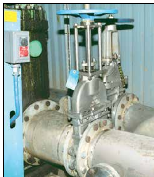
Filter isolation installation.
