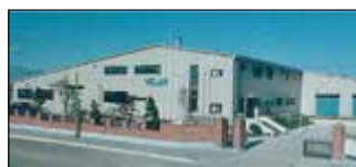
Ansan City, South Korea Velan Ltd., Plant 1
