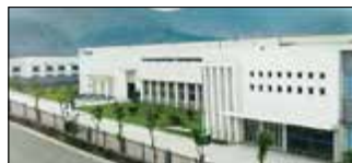
Suzhou, China Velan Valve (Suzhou) Co., Ltd.
