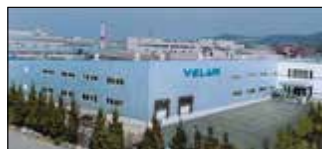
Ansan City, South Korea Velan Ltd., Plant 2
